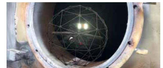
Elios drone inspecting a confined space.
