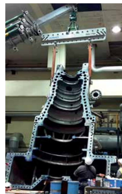
Performing a challenging turbine overhaul in Germany.
