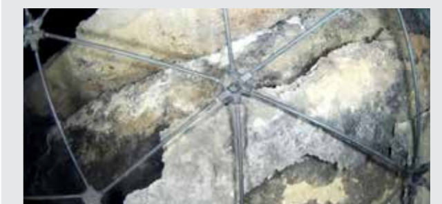
Ball drone in confined space
